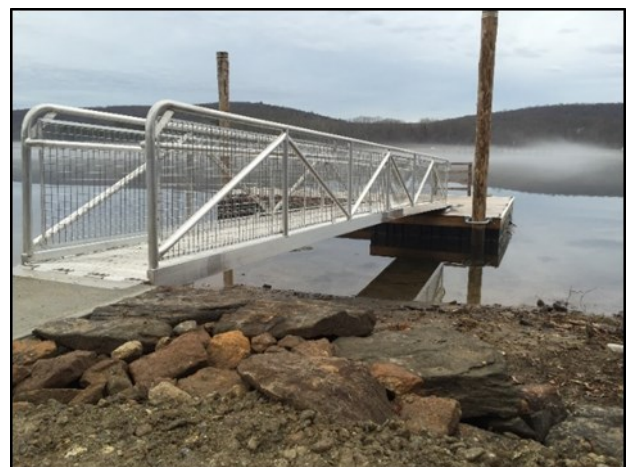
Gangplank to new town dock on the Connecticut River
