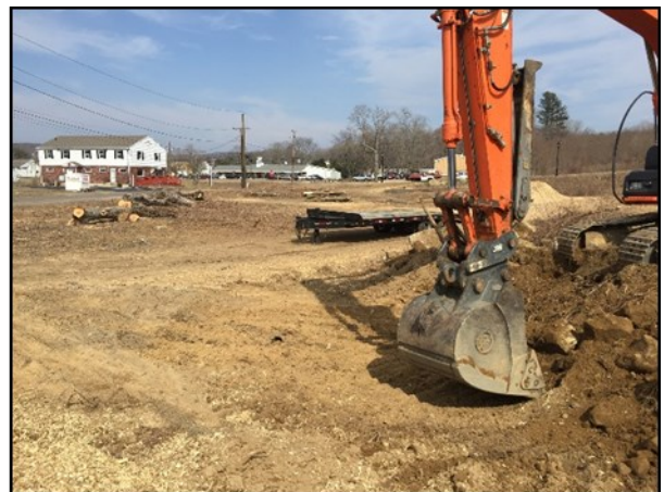
Moodus Village preparing land for commercial development
