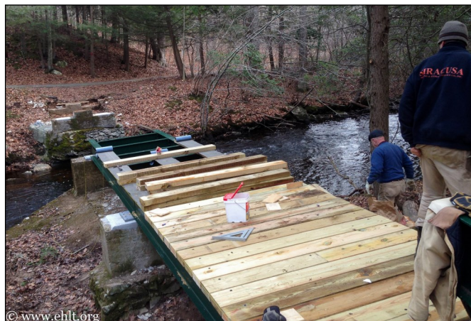
Eightmile River footbridge decking December 2015
